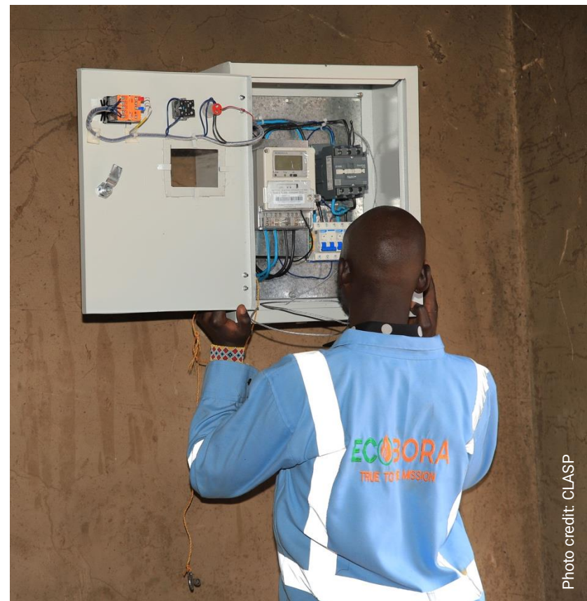
A technician installing a control box for an e-cookstove.
