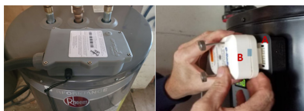
FIGURE A.3: (LEFT) Retrofit DR hardware installed on an electric resistance water heater. (RIGHT) A CTA-2045 compliant communications module, denoted as 'B' is plugged into a CTA-2045 compliant port, denoted as 'A', on a heat pump water heater. Note that CTA-2045 ports are also able to be plugged into electric resistance water heaters. Source: Sukow, "Wireless Functions Add Value to Armada Power Water Heater Control."
