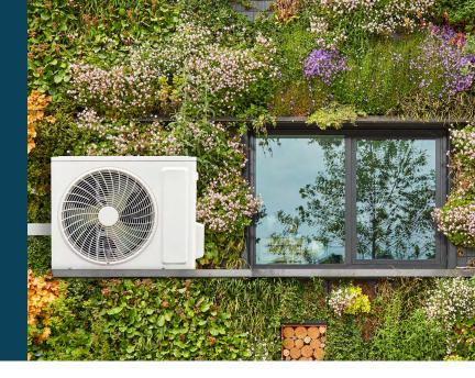
Heat pumps are highly efficient solutions for space heating and cooling. When it comes to heating, they're three to four times more efficient than electric resistance heaters which convert electricity into heat at 100% efficiency. Heat pumps are also far more efficient than the most advanced gas heating systems, which operate at only 85-99% efficiency.
