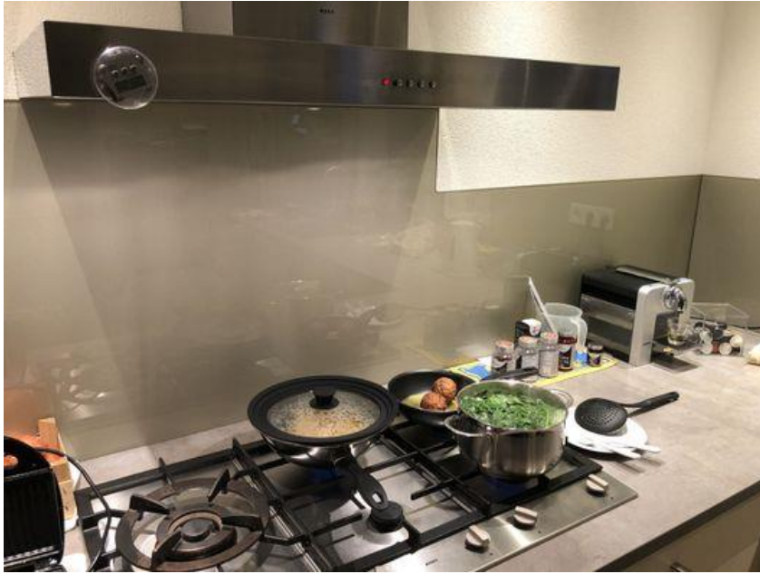
Figure 4.9 example of an effective range hood covering all burners.
