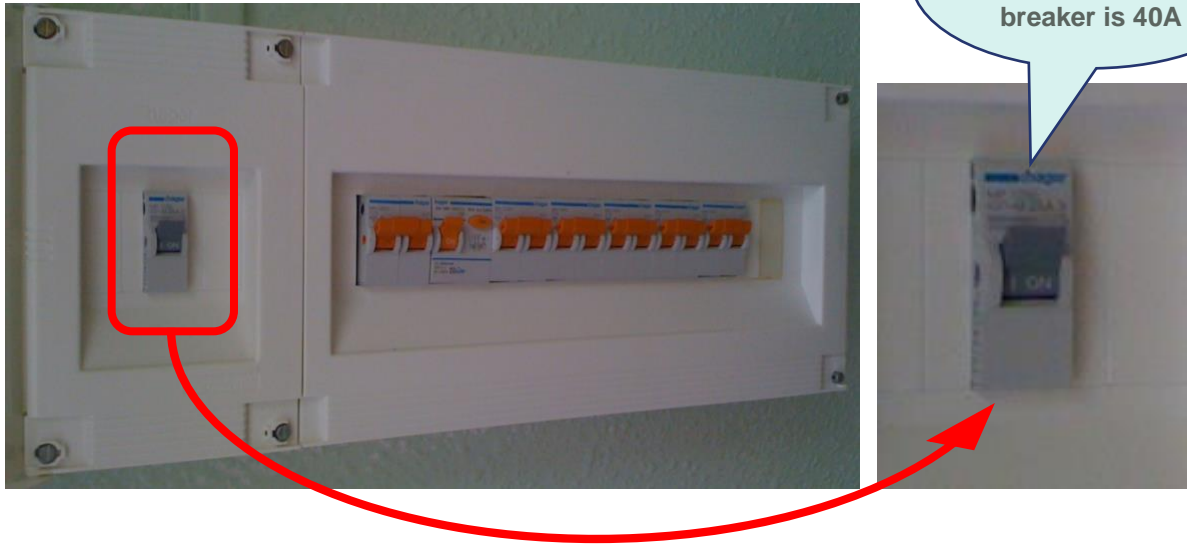
Example 3. Circuit Breaker Box and Close-Up of the Main Breaker
