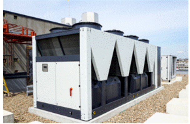
FIGURE 4 TYPICAL AIR-COOLED CHILLER
