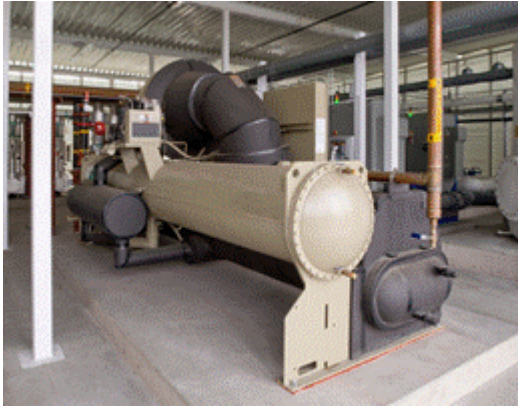
FIGURE 3 TYPICAL WATER-COOLED CHILLER
