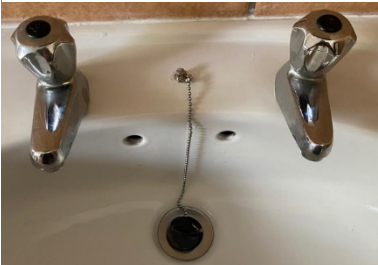
FIGURE 3: EXAMPLE OF A SEPARATE HOT AND COLD WATER TAP IN SOUTH AFRICA
