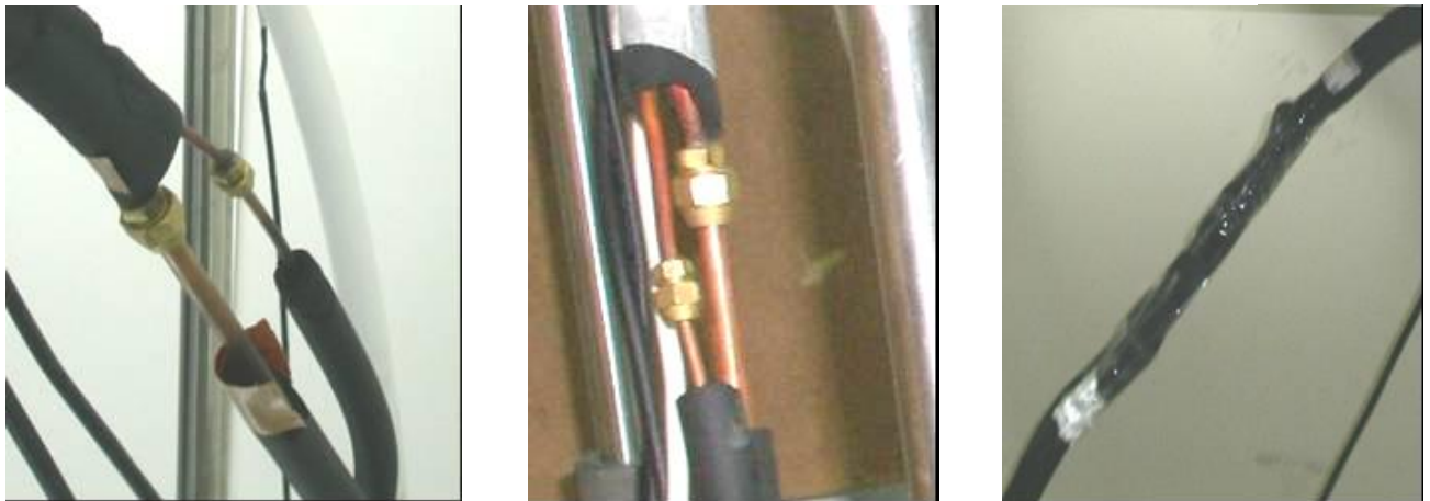
Figure 5 Refrigerant Piping Without and With Thermal Insulation
